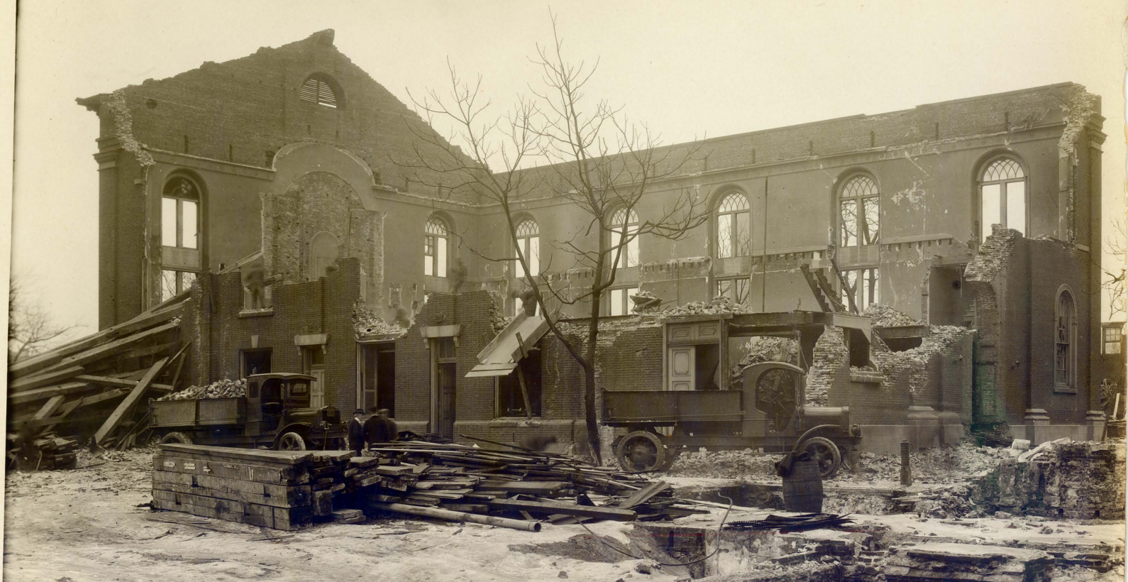
2014 Demolition of St. John's Church - Phila. 1-19-25
