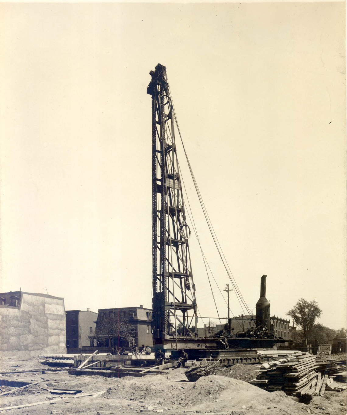
2154 Camden Approach - Pile Driving West of 4th St. 4-23-25
