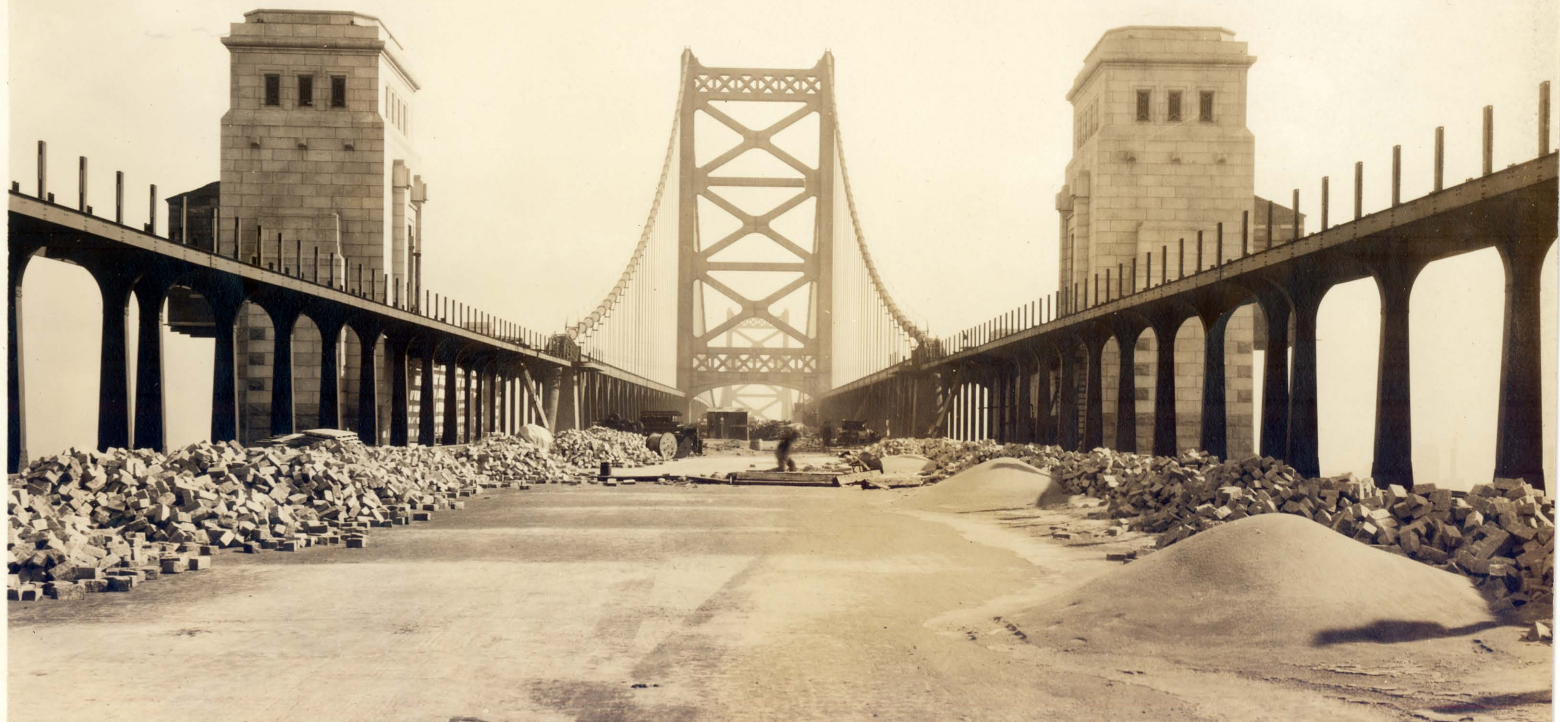
2488 Bridge Roadway Slab-Looking East from West of Phila. Anchorage 2-15-26
