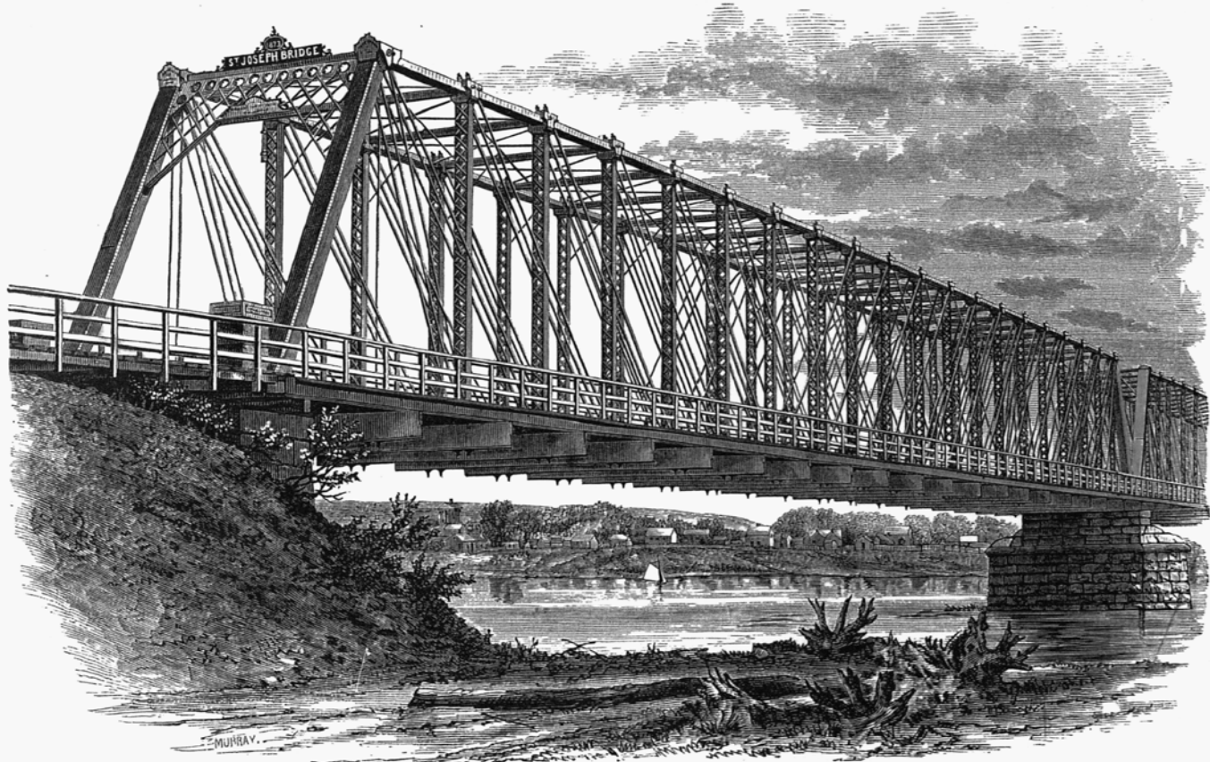
HIGHWAY AND RAILROAD BRIDGE, 250 FEET SPANS, ST. JOSEPH, MO. BY THE DETROIT BRIDGE AND IRON COMPANY.
